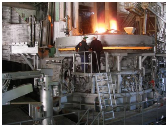
CUPTOR CU ARC ELECTRIC
